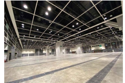
Replacement of Exhibition Hall
